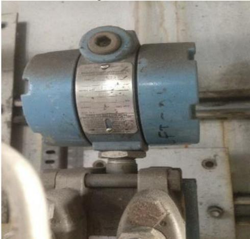
Gambar 2. *Pressure transmitter*
