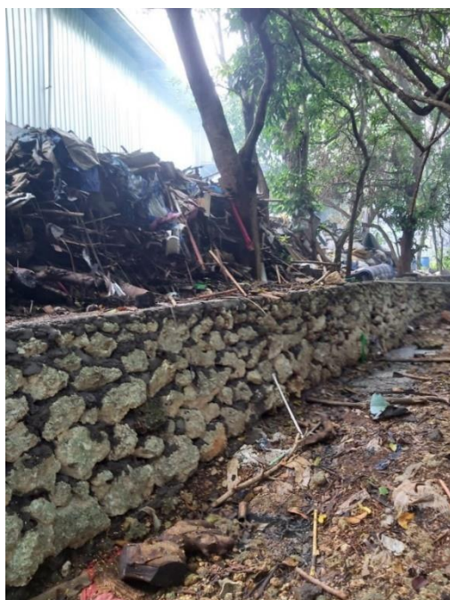
Figure 5. Rubbish spilling into the creek January 2022
