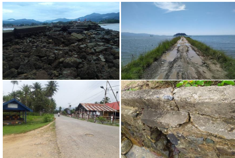
Figure 1. The existing condition of Tinobu Port Field Survey Data
