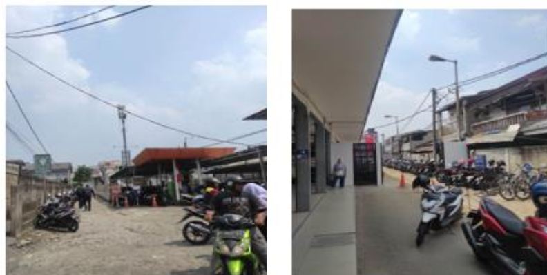
Figure 3. The existing condition of parking at Depok Lama station
