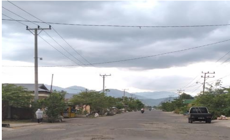
Figure 4. Condition of power grid in Kobo Kecil village Source survey in 2023
