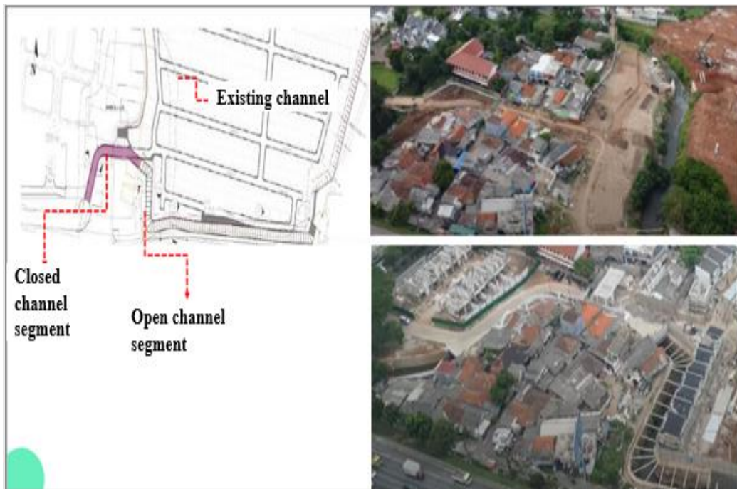
Figure 3. Overview of the Channel Diversion Project. Source: Project Processed Data 2023
