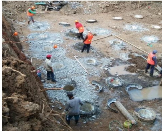
Figure 2. Pile Breaking
