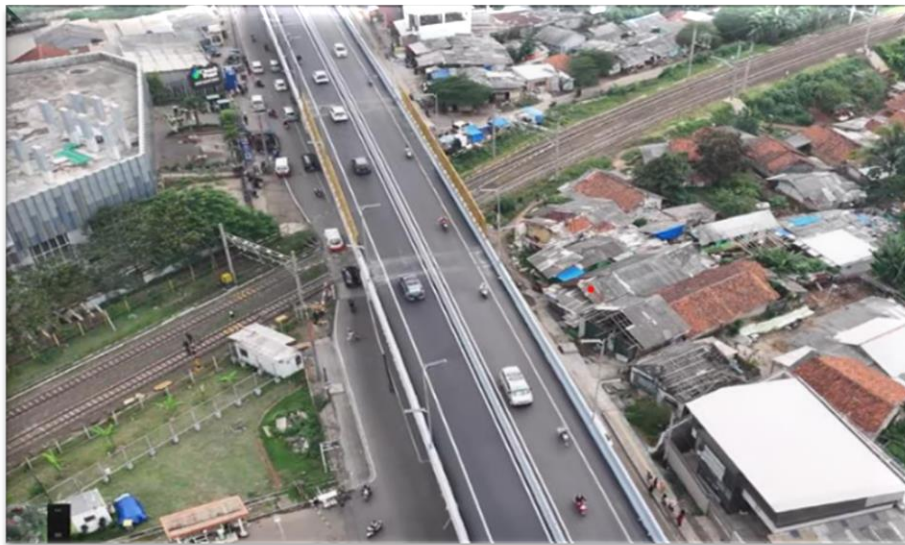
Figure 2. Final Condition of Work (Source: Project Processed Data (2023))
