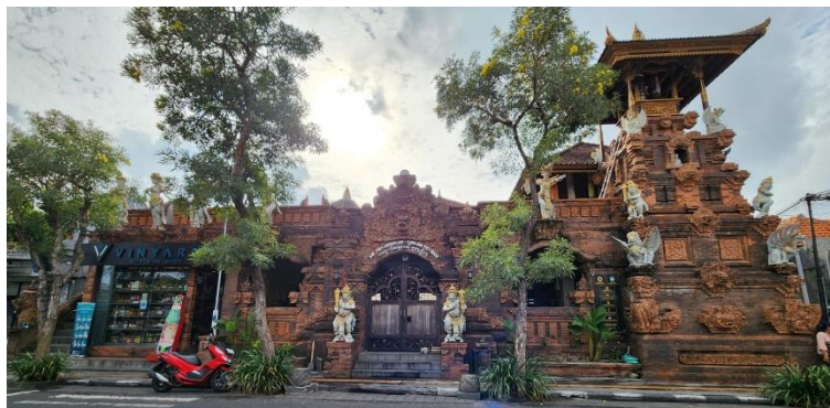
Figure 2. Bale Banjar Pekandelan Legian, the ground floor is also rented out for a shop
