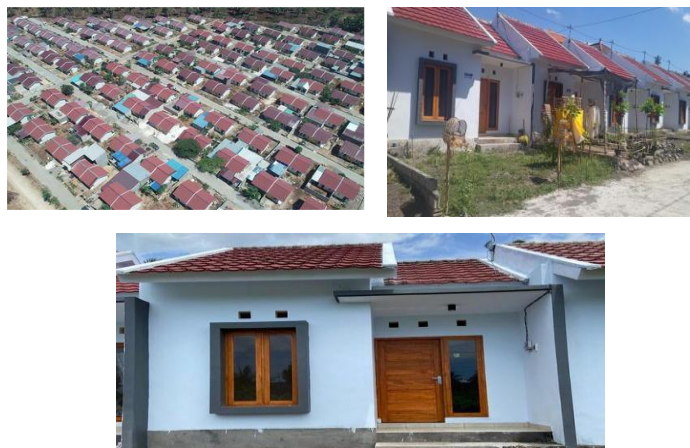
Figure 2. D'Gedong Residence Housing
