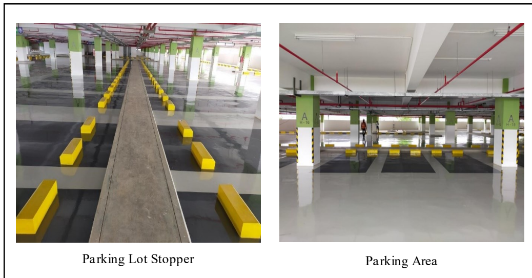
Figure 1. Existing Condition of Sultan Hasanuddin Airport Parking Building
