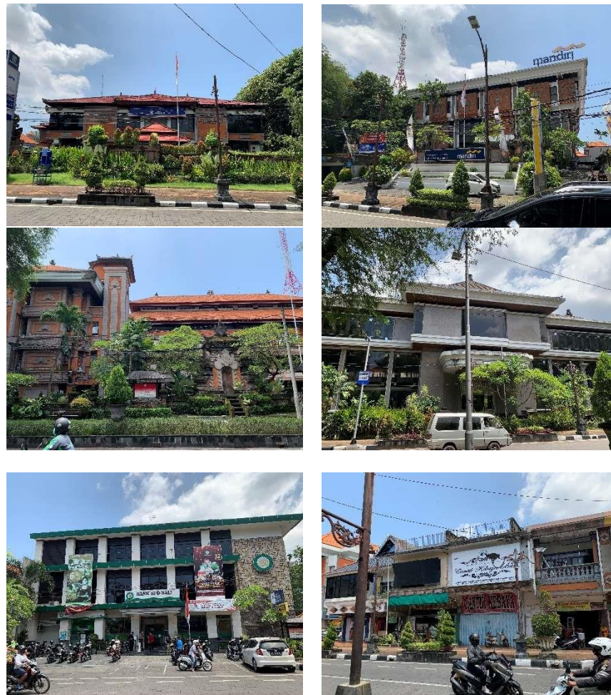
Figure 6. Building facade Segment 3
