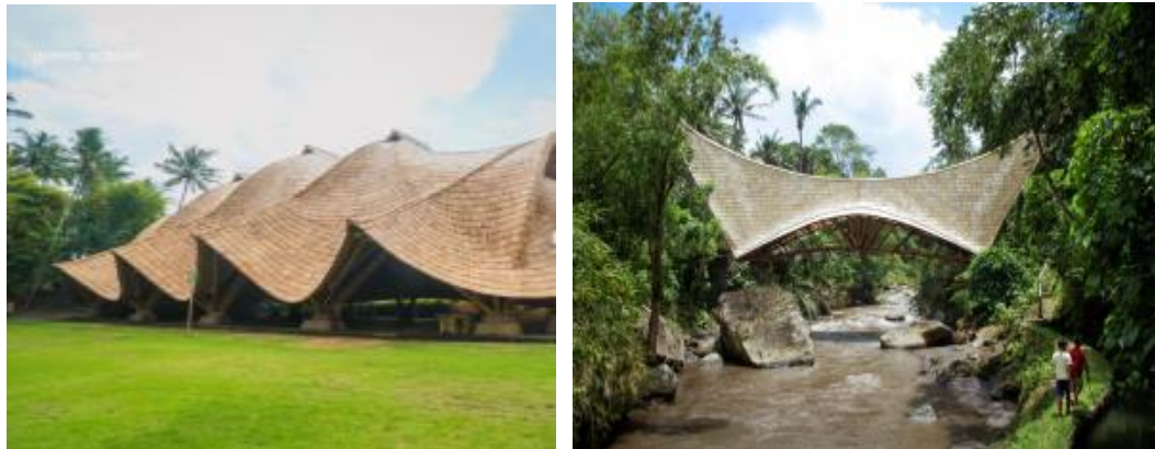
Figure 5. the arc and bridge of Minang Green School Bali. Source : Instagram @greenschoolbali , 2022
