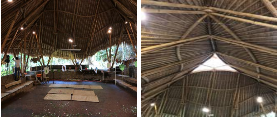
Figure 9. Openings and skylights in the Green School Bali performance space. Source: Personal Documents, 2021.
