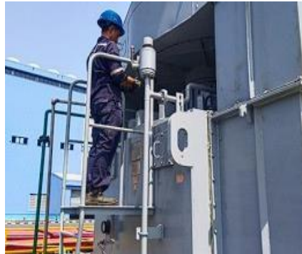
Gambar 3 Pengukuran Insulation Resistance
