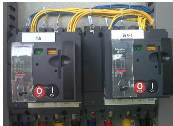
Gambar 5. Motorized Air Circuit Breaker (ACB)
